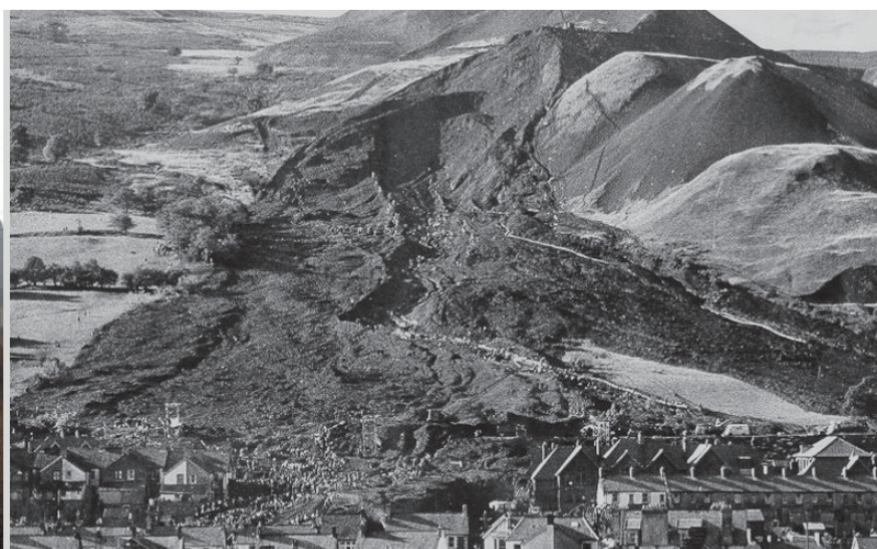
1966 collapse of a coal-gangue tip in Aberfan, Wales, U.K., which killed 144 people, including 116 children
