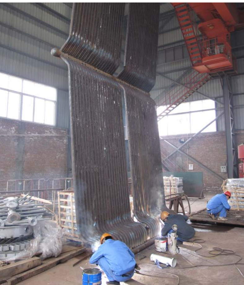
Manufacturing of one the brick kiln roof heat exchanger components
